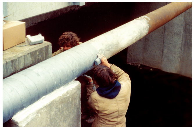
Here Trenton's Wax-Tape® #2 wrap is being applied over the Wax-Tape® primer (white). Notice that the Wax-Tape® primer can be applied to the pipe after only minimal surface preparation.
