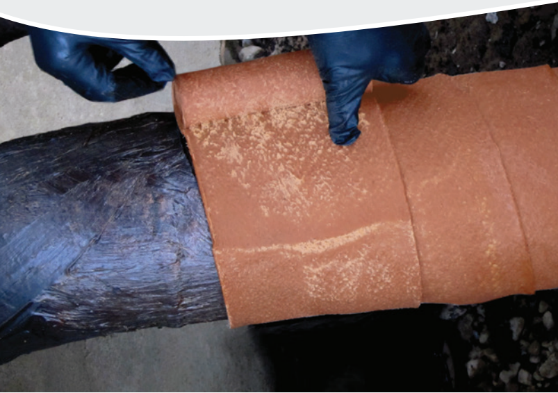
An easy-to-apply protection system for high-temperature applications, Wax-Tape® HT-3000 wrap requires minimal surface preparation.
