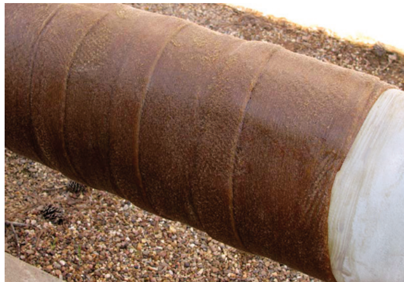
After coating with primer, the wrap should be wrapped onto the pipe in a spiral pattern using a minimum 1" overlap. Seams and ends should be sealed.
