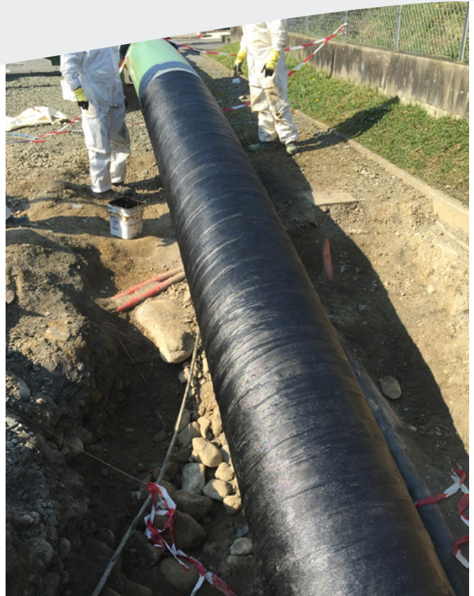
Transition areas are hard to protect against corrosion and mechanical damage, so the MCO™ 110 outerwrap and Wax-Tape anticorrosion wrap combination provides an important resource for corrosion engineers.
